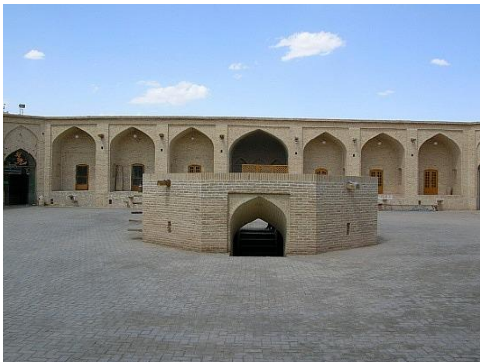
View of a renovated caravanserai
